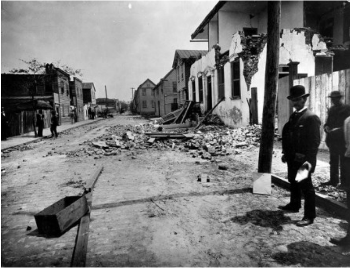
William John McGee of the U.S. Geological Survey inspecting a fissure near a wrecked brick house on Tradd Street in Charleston. Photo by John Karl Hillers, USGS (public domain).
